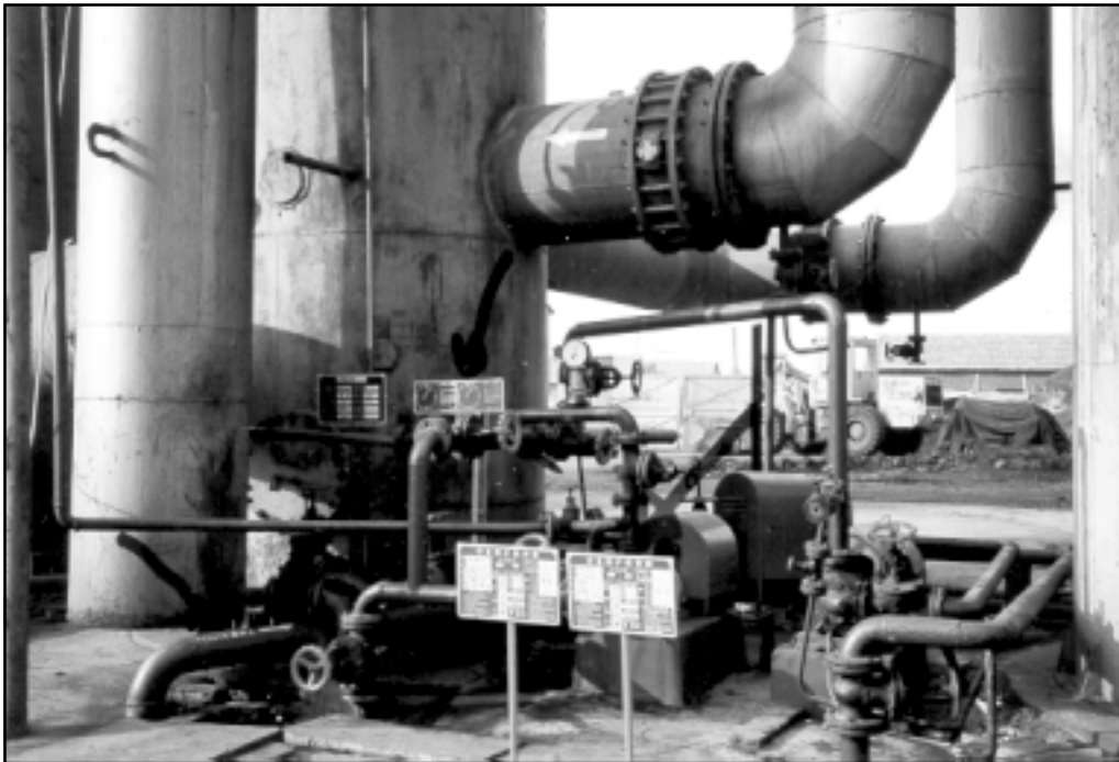
In this factory in Fuyang workers used Good Housekeeping techniques to correct leaking valves and other equipment problems, resulting in reduced exposure to ammonia fumes.
