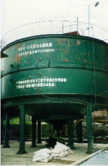
Photo 17: White water flotation basin
