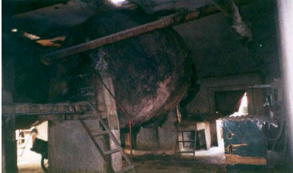
Photo 3: Steam injection in digesters
